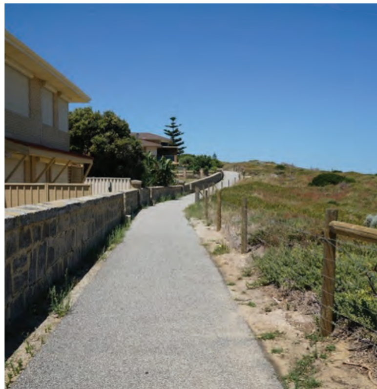
Figure 363: Shared path running between foreshore reserve and private residences.
