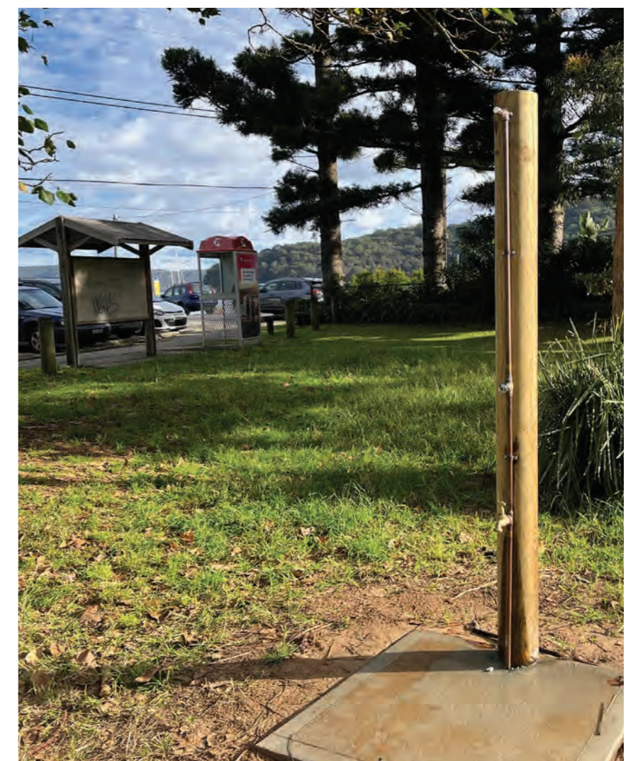
Figure 344: Old showers at Patonga Beach.
