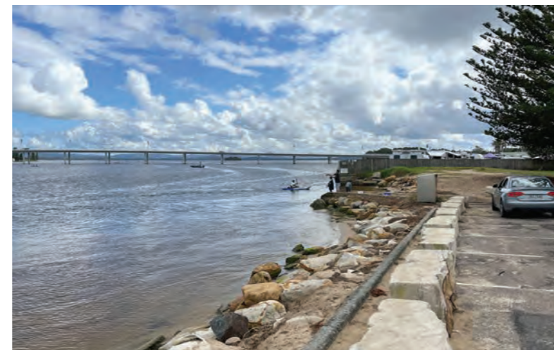
Figure 358: Seawall on the north side of The Entrance Channel.
