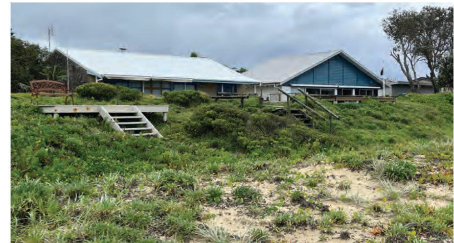
Figure 360: Private access to Hargraves Beach, including stairs and viewing platforms.
