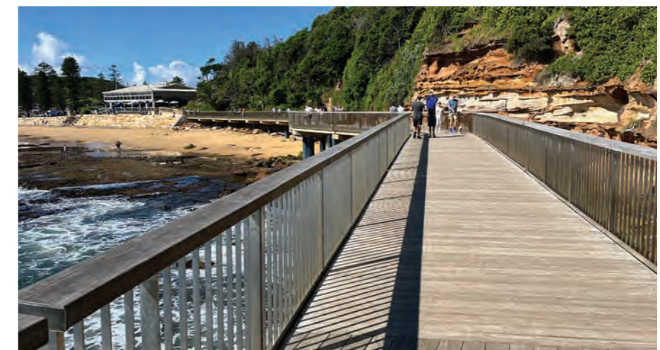
Figure 280: The Terrigal Haven Boardwalk forms part of southern section of the Terrigal Beach path.
