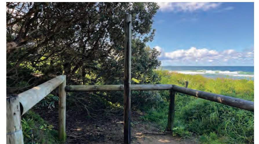
Figure 319: Another old shower at North Avoca Dog Beach at the end of Lake Street.
