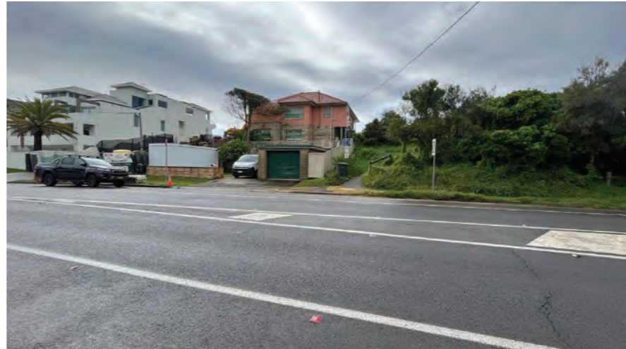
Figure 386: Local access point on Ocean View Drive south of Lake View Road junction.
