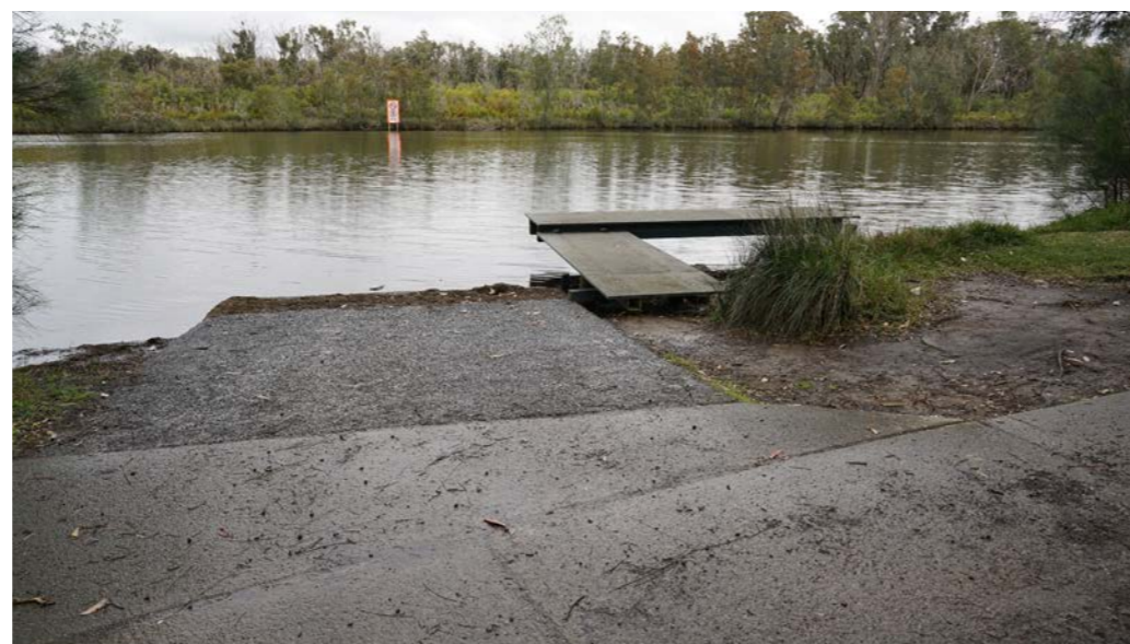
Figure 59: The small jetty and boat ramp at Brudenell Avenue.
