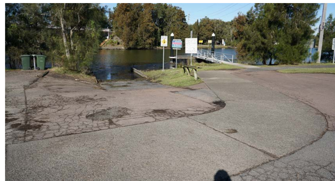
Figure 74: Budgewoi Point Boat Ramp and Jetty.
