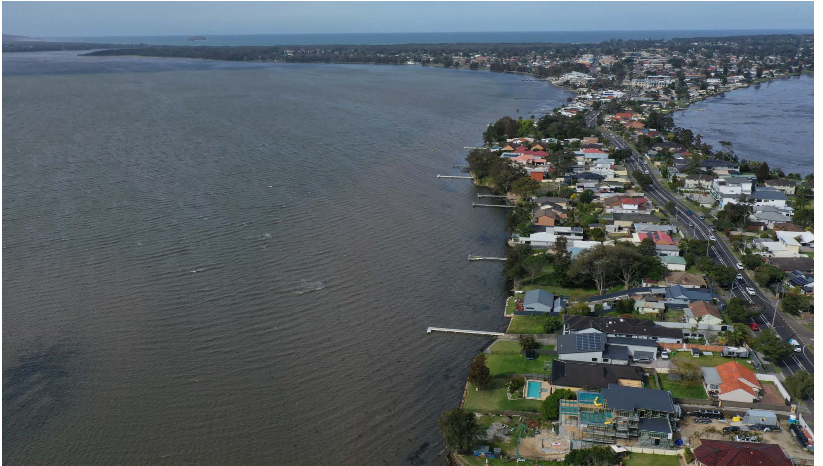
Figure 56: Looking east along Main Road Foreshore.
