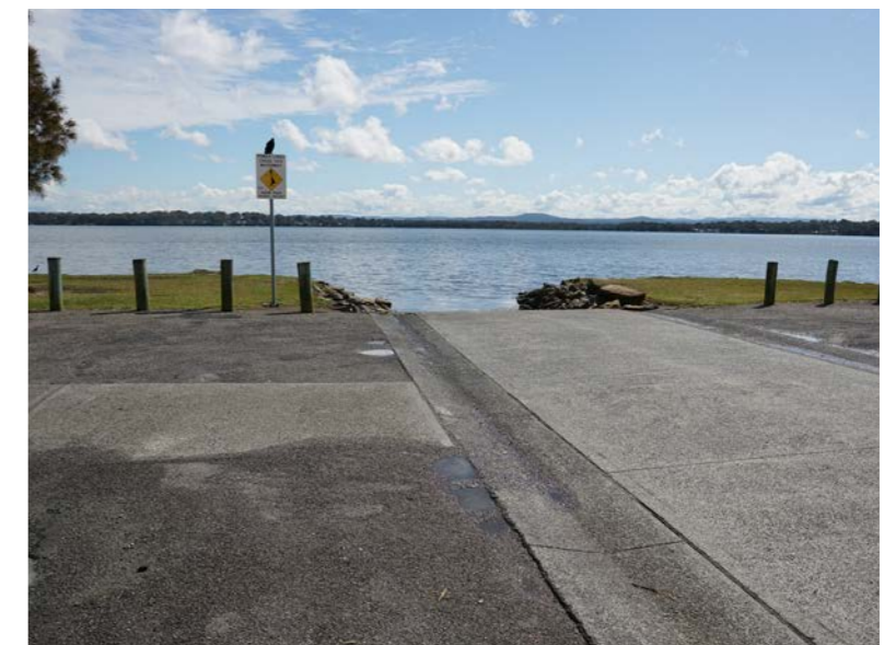
Figure 66: Boat ramp at Edgewater Park.
