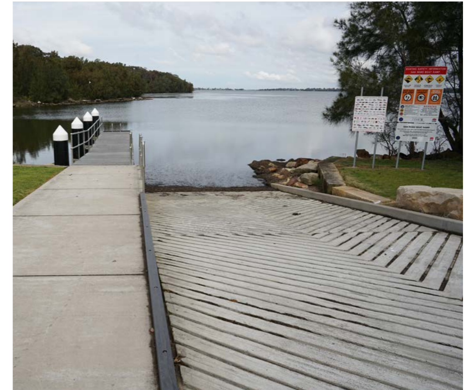
Figure 61: San Remo Boat Ramp.
