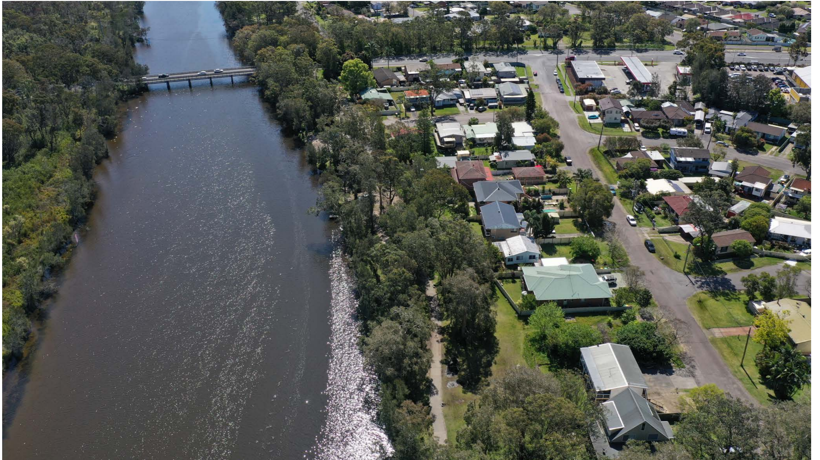
Figure 60: Looking west over the bridge across Wallarah Creek, with the start of the foreshore shared path visible through the trees, as is Brudenell Avenue Boat Ramp behind it.
