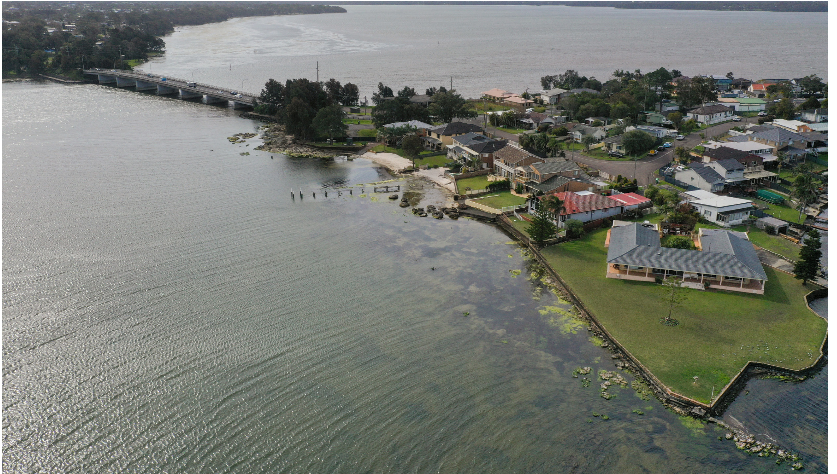
Figure 107: Looking north over Wallarah Point, with Main Road Bridge behind it.
