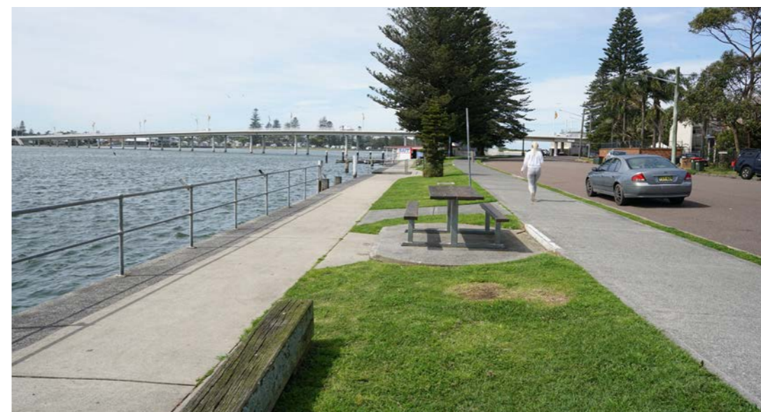
Figure 113: Looking east along The Entrance Road shared path.
