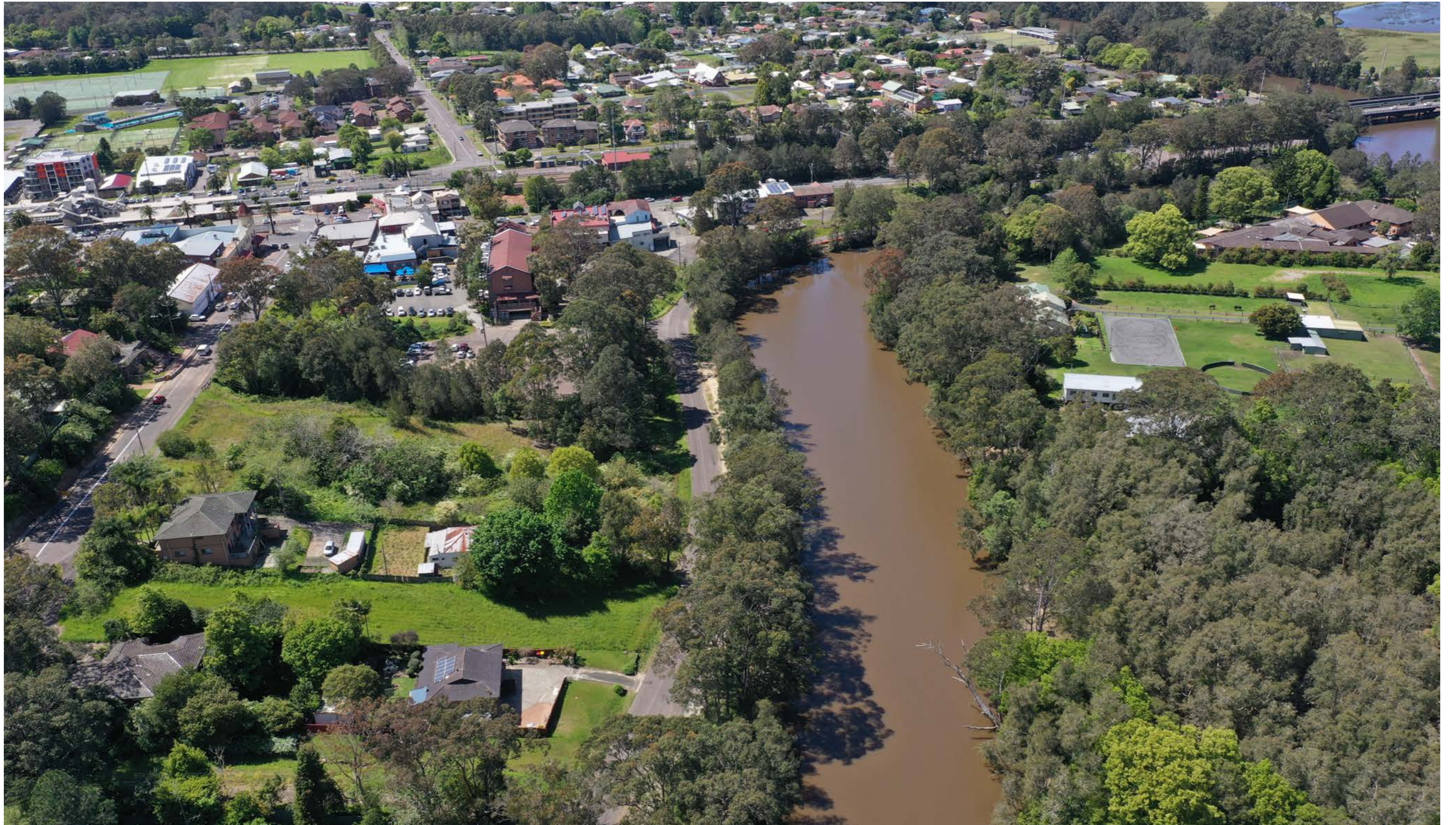
Figure 95: Looking east towards Pacific Highway: River Road Urban Connector is visible on the left bank, and the Rural Residential Connector on the right bank.
