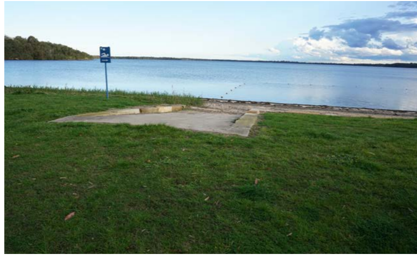
Figure 203: Lake Munmorah, Tom Burke Reserve: good facilities but boat launching ramp difficult to access.
