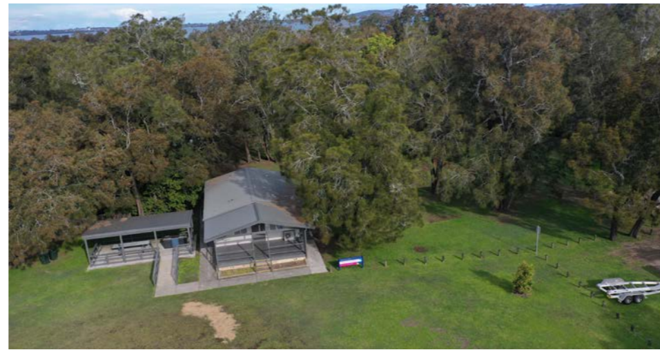
Figure 157: Facilities at Sunshine Reserve.
