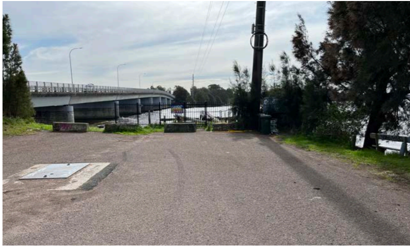
Figure 211: Tuggerah Lake, Main Road Bridge Reserve: degraded area, 4 carparking bays, bins, damaged jetty and damaged path under bridge.
