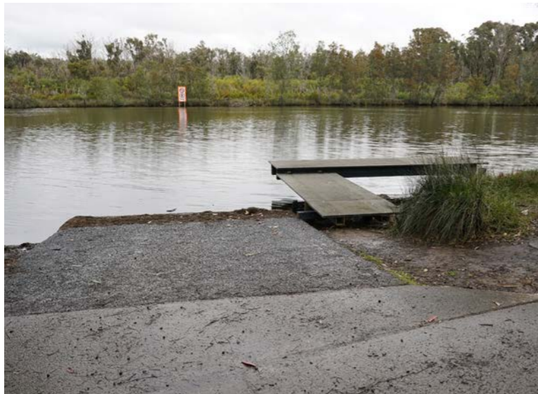
Figure 172: Brudenell Avenue Boat Ramp.
